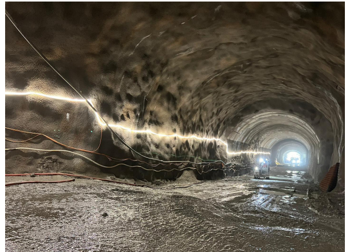
Implenia Switzerland, ARGE Gotthard
