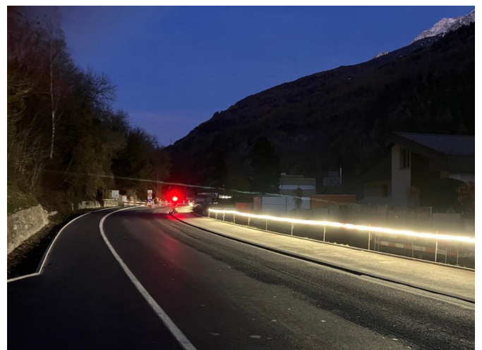
Construction site Bitsch VS
